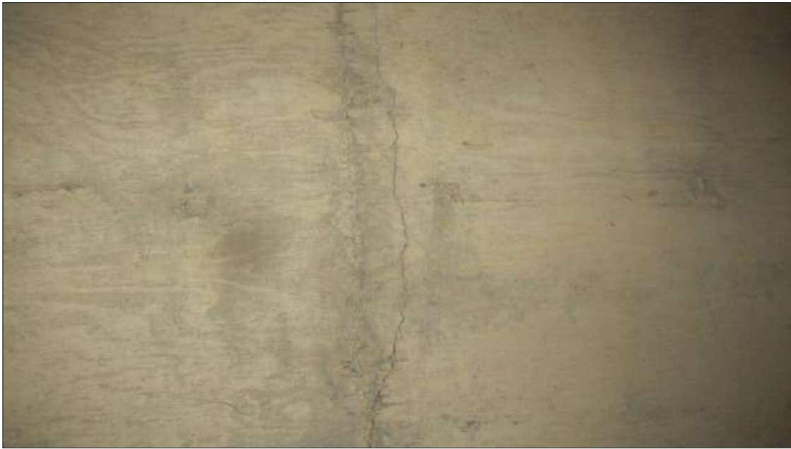
Barrel 3 Section 1: 4 Feet of Cracking (RC and Other): Width less than 0.012 in. or spacing greater than 3.0 ft. VERTICAL CRACKING
